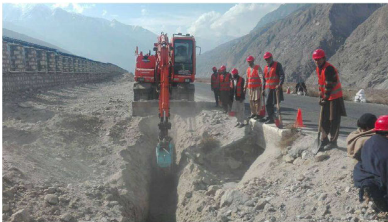
Image 10: Optical Fiber Cable from Rawalpindi to Khunjrab | Source: cpecinfo.com
