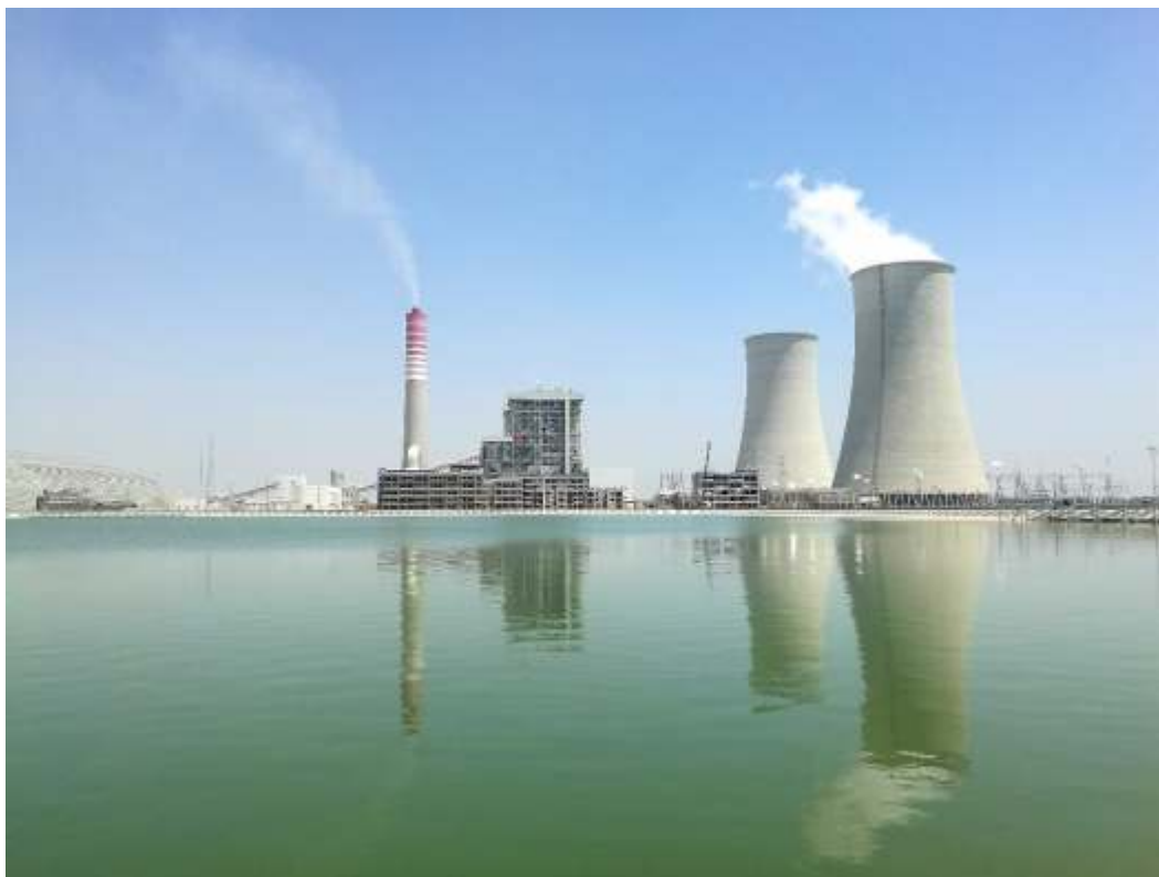
Image 3: Sahiwal Coal-Fired Power Plant, Punjab | Source: cpec.gov.pk
