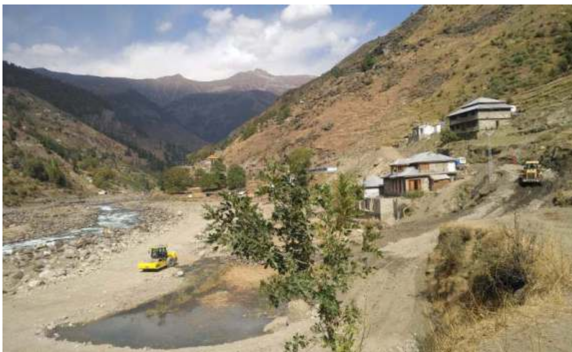
Image 5: Suki Kinari Hydropower Station, Naran, Khyber Pakhtunkhwa | Source: cpec.gov.pk
