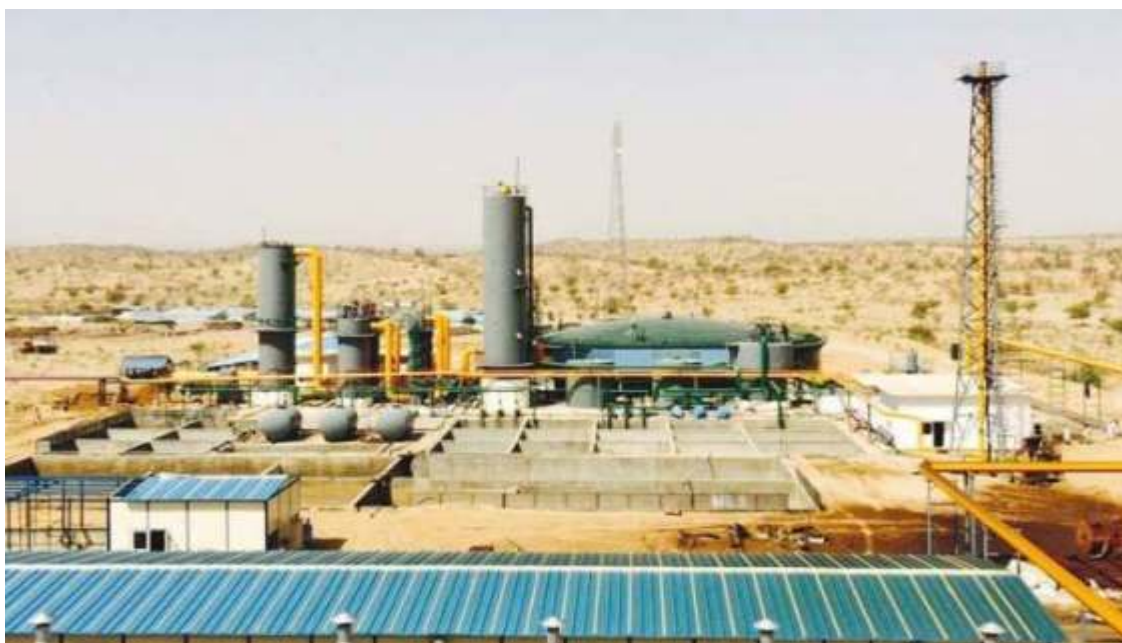
Image 12: Engro Thar Block II Coal Fired Power Plant, Sindh | Source: cpec.gov.pk
