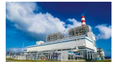
Overall View of CPHGC
