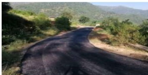
New Constructed Access Road in Hollar
