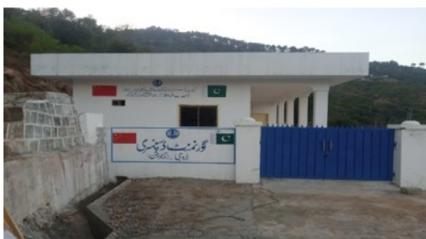
A view of new dispensary building at Brohi
