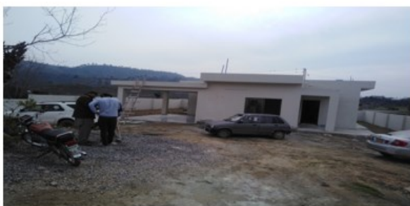
Newly constructed rest house in Beor
