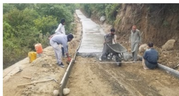
Construction of Access Road Kahutta
