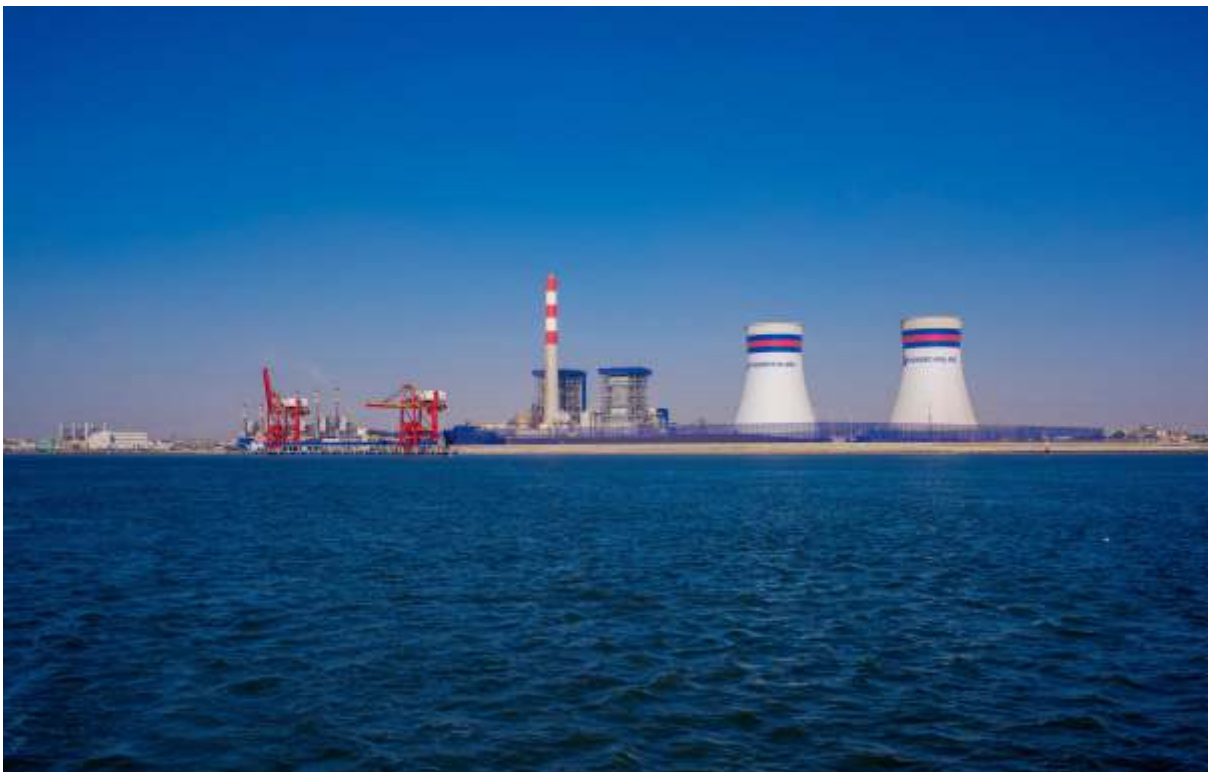
Blue ocean and “1,320 MW (Super Critical Technology) Port Qasim Coal-fired Power Plant
