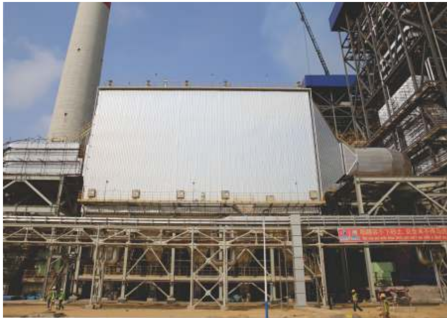
Figure 2 Electrostatic Precipitator
