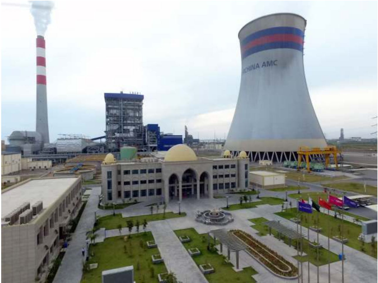
Green and Clean atmosphere with “1,320 MW (Super Critical Technology) Port Qasim Coal-fired Power Plant”
