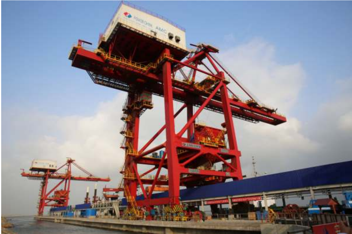
Figure 8 Complete view of in-house “Coal Unloading Jetty and Covered Conveyor Belt”
