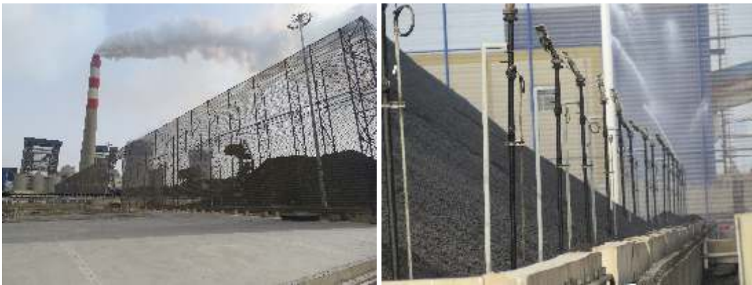
Figure 11 Wind Breakers and Water Sprinklers across the coal yard
